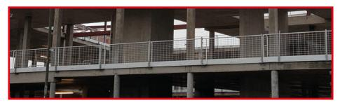
Altrad Generation provides edge protection solutions for concrete frames including systems that don't require any penetrating into the concrete at all. The Rapid Post is a telescopic post that offers single, extended and full containment edge protection using very few components which vastly reduces the installation process.
