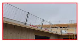
Altrad Generation provides a full range of components for hire for the timber frame edge protection. Like with our steel frame edge protection, you can install our components for Timber Frames on the ground making installation safer and more efficient. We are also able to supply you with top fix solutions and side fix solutions and handrails or mesh barriers can be used.
