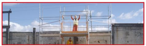
Genlok can be used to create Loading Towers for the purpose of distribution of pallets of materials to the working level by site forklift or loader.
