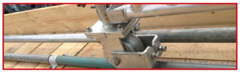
The purpose of the Trax bracket is to provide a cost effective, quick and efficient method for rolling out beam assemblies, gantries or temporary roofs.
