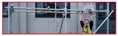
Altrad Generation Readylok Transom units will, at low cost immediately convert your stock of tube and fittings into an easily and speedily erected system scaffold, whilst maintaining TG20 compliant. The use of these pre-coupled units dramatically eliminates the need for loose fittings. In use they will considerably speed erection times reducing labour cost and site losses.
