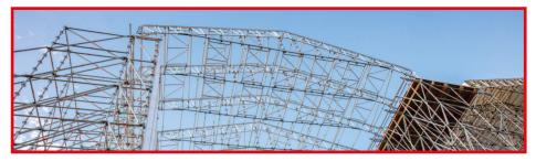
The use of innovative intermediate roller brace coupler makes split bays very easy to achieve together with the deeply-shrouded track spigot; this has previously been difficult if not impossible with Keder-style roof coverings.
